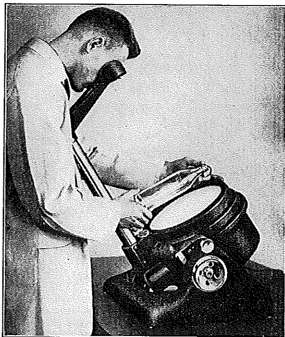
FIG. 11.—Polaroid polariscope.
